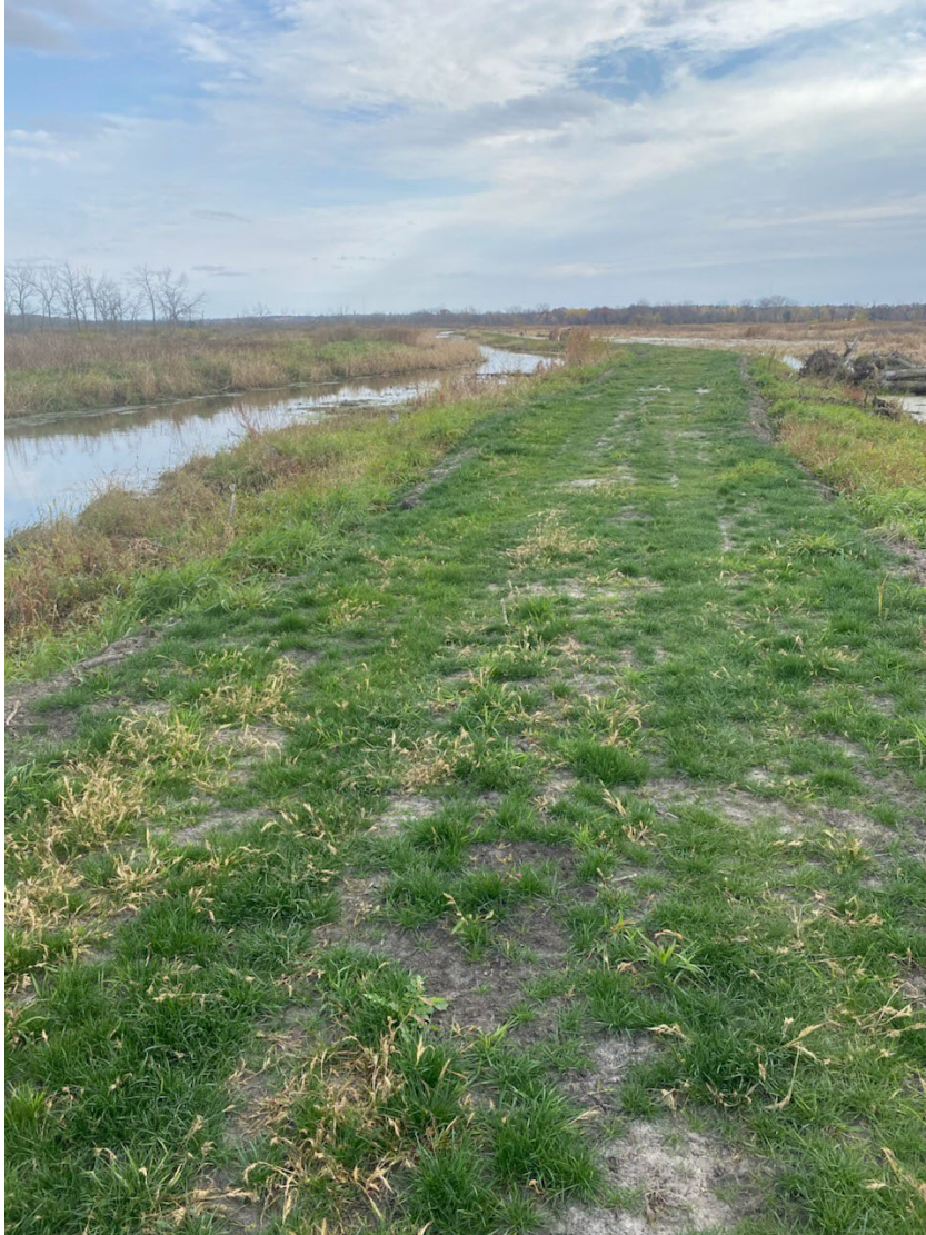
Final project stabilization Annual Inspection of Town Drain
