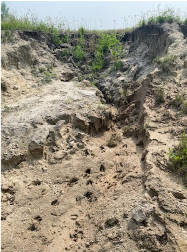
Project before repair, spring 2026
