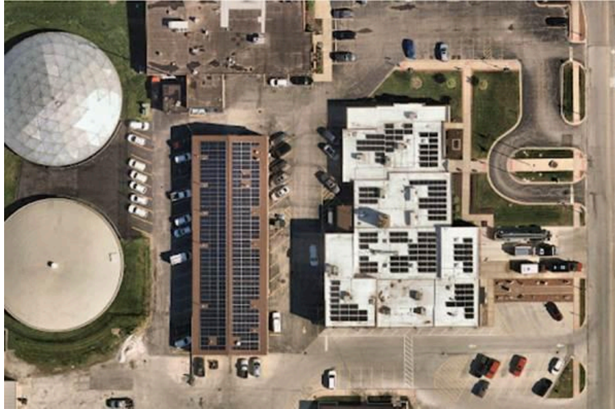
Figure 3: Village of South Holland municipal solar installation.
