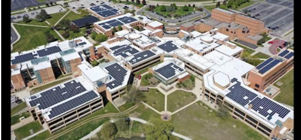
Figure 4: College of Lake County ground-mount and rooftop array.
