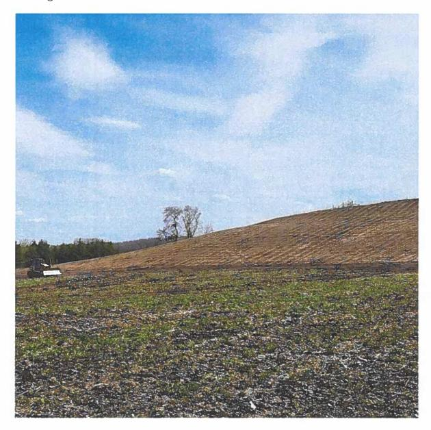
Note. Slopes have been finish graded and seeded, floor prep in progress.
