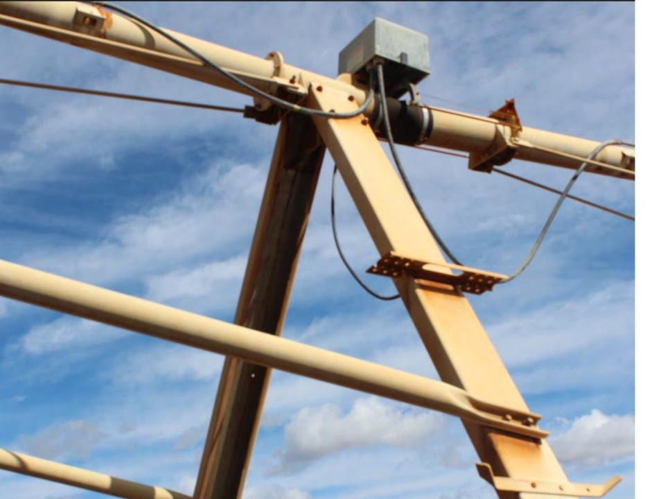
With only 106 hours of pumping the water stripped all the galvanizing off the brand-new center pivot irrigation equipment. This was caused by sulfide s in the Platteville and St Peter being oxidized as acid mine drainage reaction.
