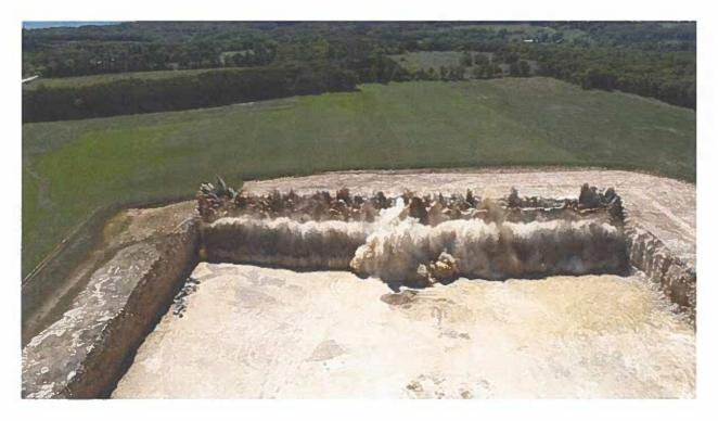
Note. The last hole has detonated by this point.
