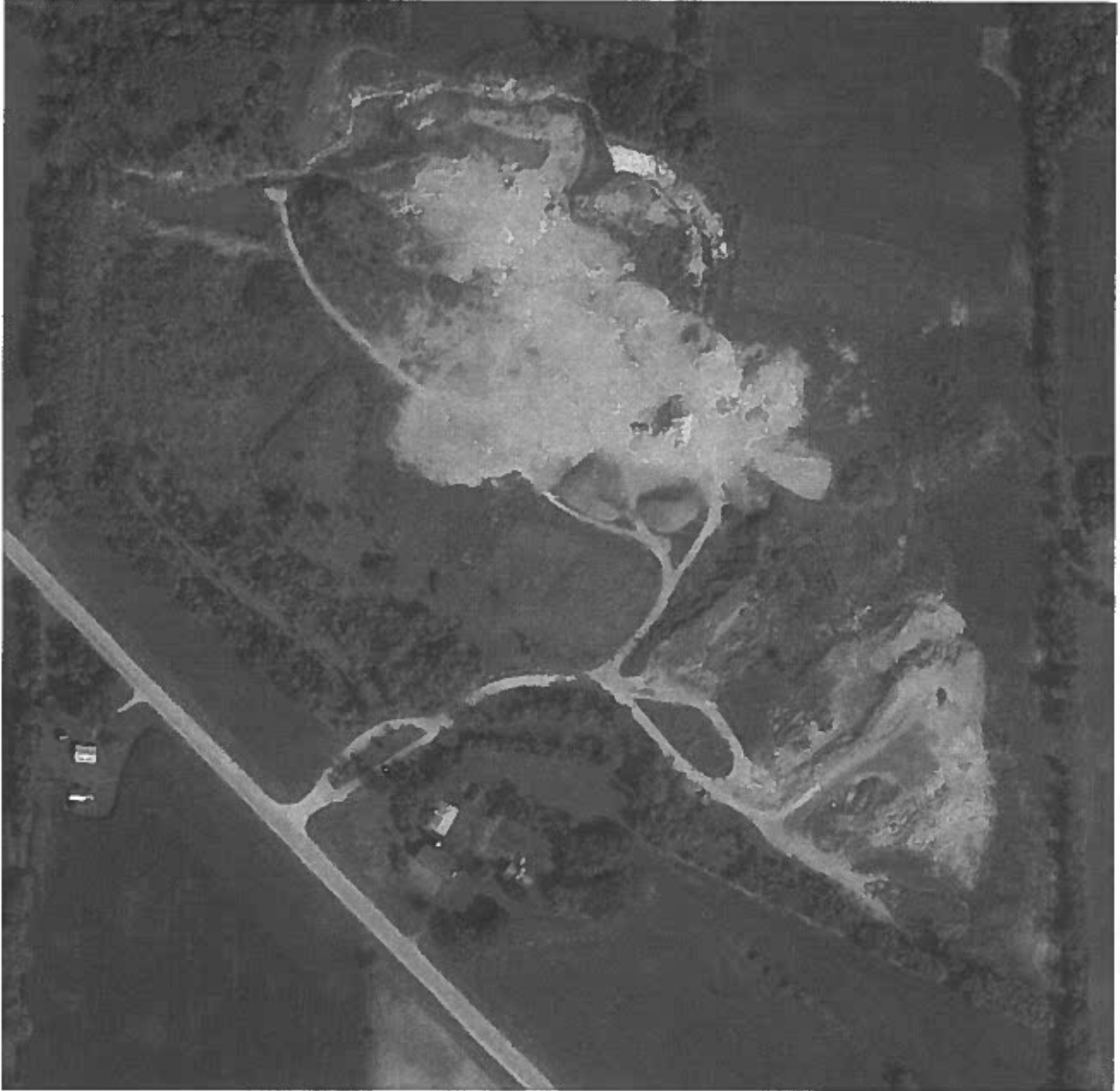
Note. Reclamation progressing. 2017
