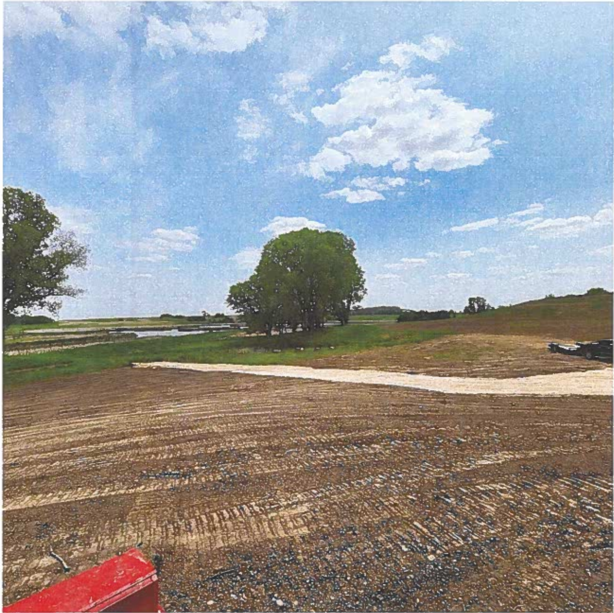
Note. Floor has been seeded.
