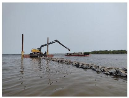
Construction was scheduled for spring of 2023 with large barges that could complete the project within 3-4 weeks. Construction began May 1<sup>st</sup> and was completed by the end of the month. The project entailed placing more than 9,000 tons of rock on top of the existing dredgebank, covering 3,000 feet of restoration.
