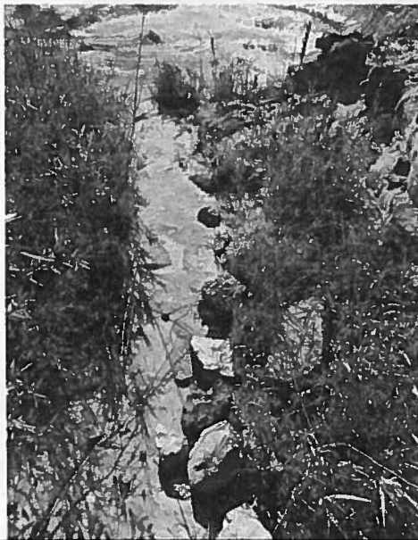
View of past water intrusion location in Area 2
