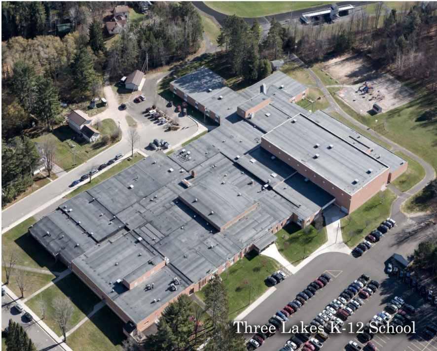
Three Lakes K-12 Elementary School
