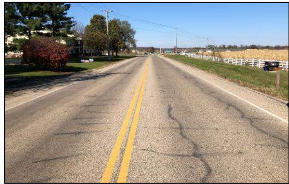
Figure 5 –South of South St/Sunnyside Rd
