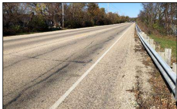
Figure 7 – South of Structure B-24-005
