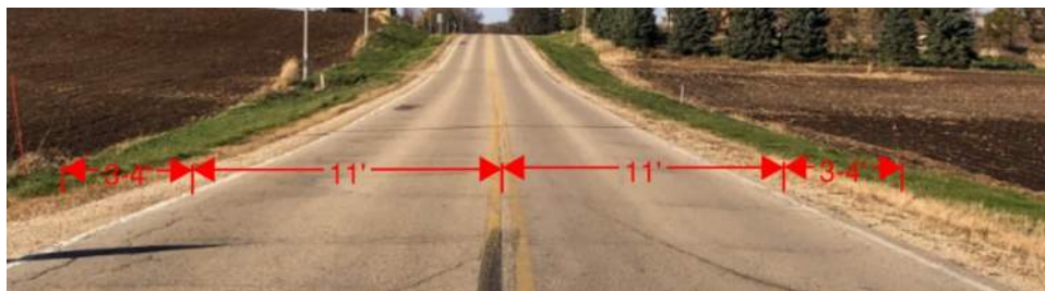
Figure 9 – Existing Typical Section For Final ~2,000'
