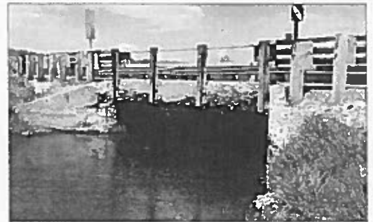
Existing deteriorated structure. Water has overtopped the structure recently.
