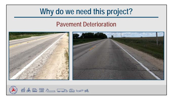
This project is needed to address the pavement deterioration along County A. The existing pavement is aged and deteriorated with extensive alligator cracking, edge cracking and patching, and transverse cracking, resulting in a rough riding surface.
