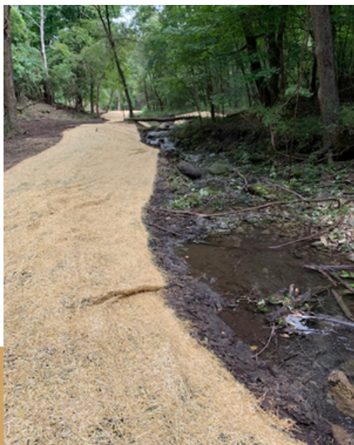
Streambank right after the restoration.
